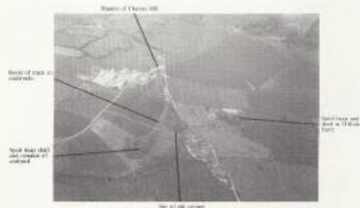
Fig. 3. Aerial view showing disused coalmines
