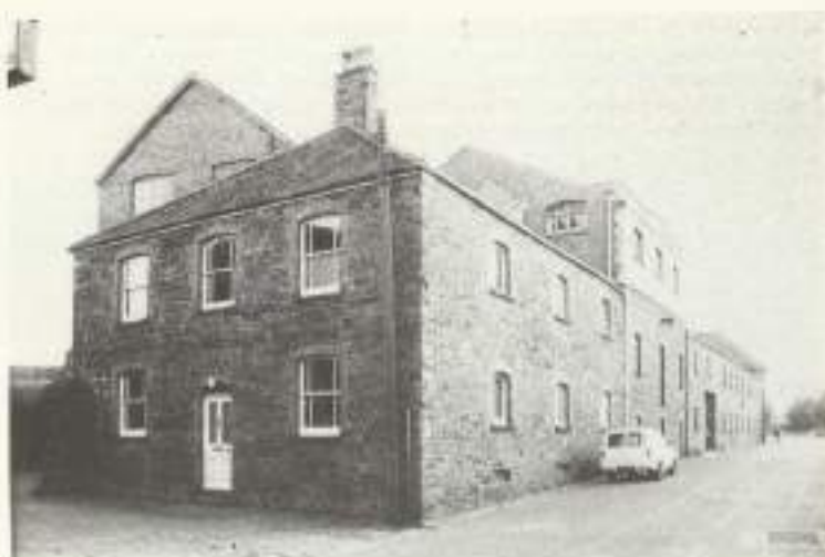
Plate 1. Lodway brewery, front view from east, in 1980.
